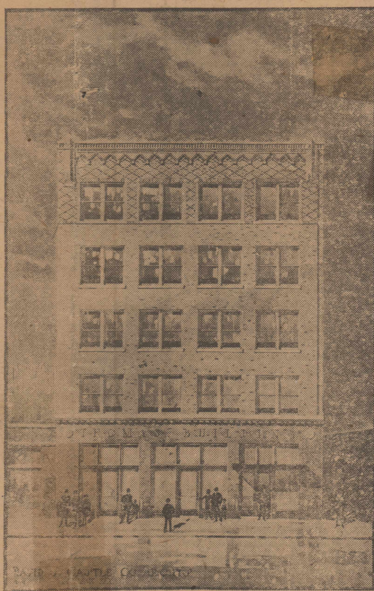
The new Thomas office Building
