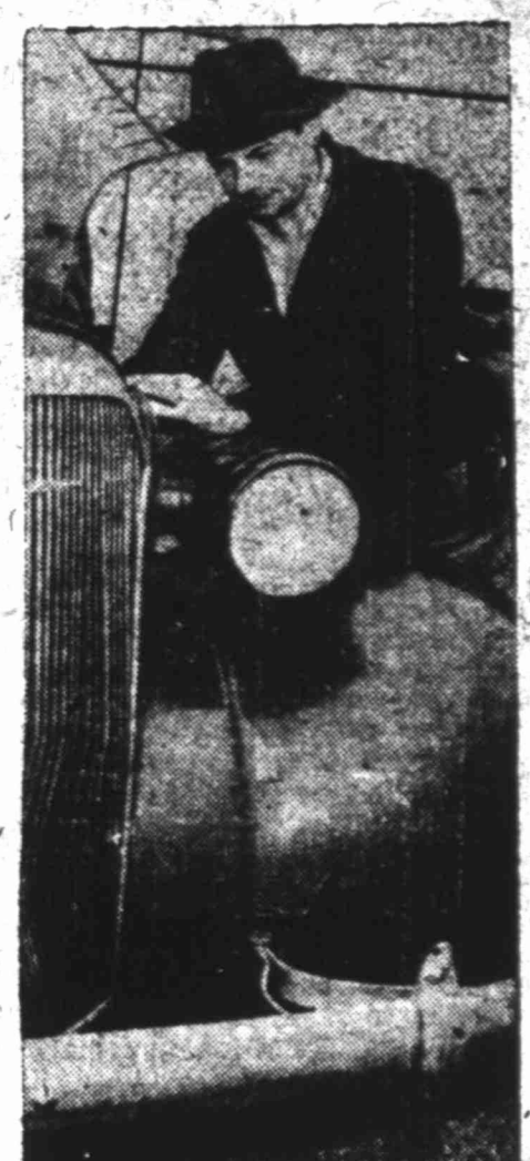
Floyd Kupchik makes repairs.
