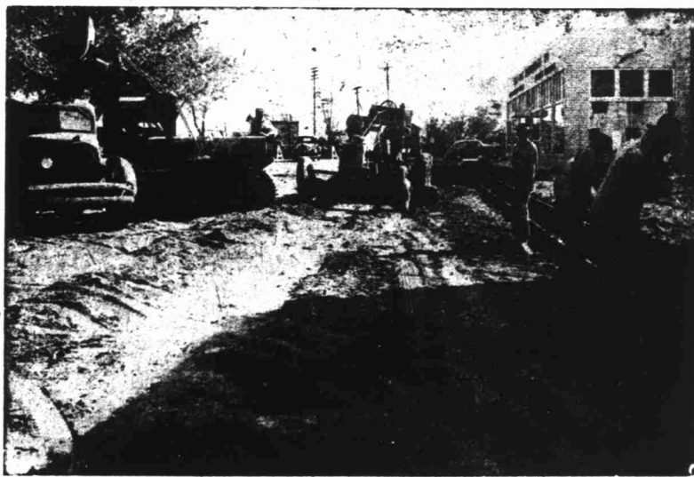
The picture shown above was made at the start of the Midland paving program. This paving was laid on North Ft. Worth Street . . . experienced men and modern equipment were required to do this job.
