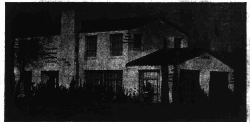
Williamson Home—Roofing Work by Shepard Roofing Co.
