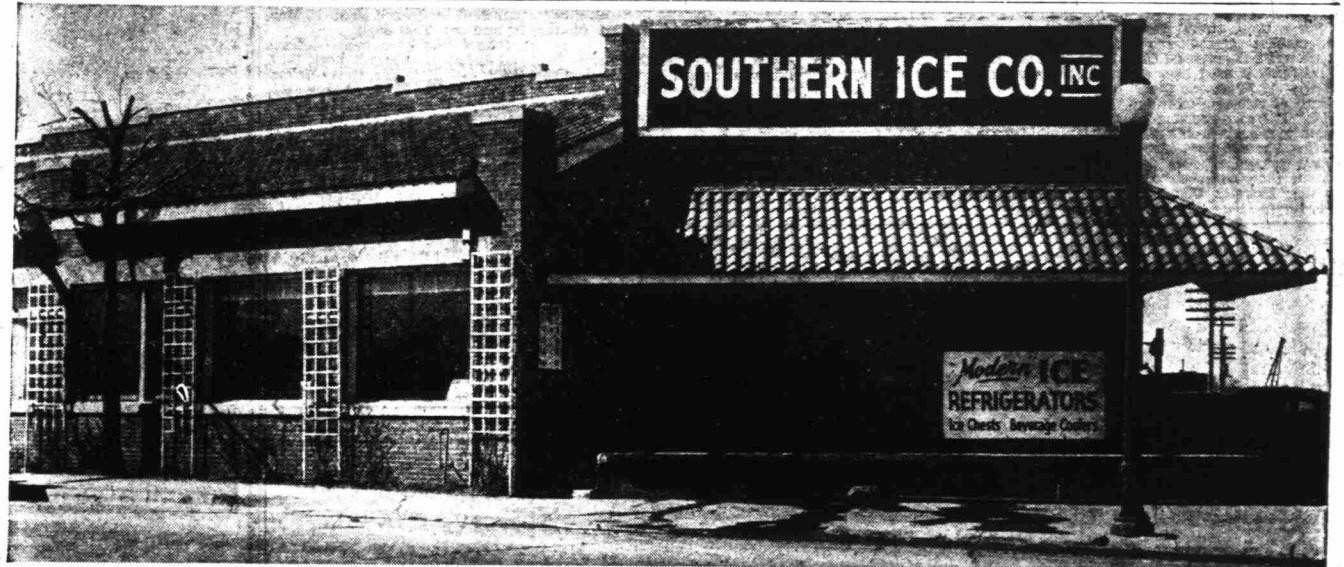
For 21 years, the trucks of Southern Ice Co., Inc. have been faithfully serving Midlanders with quality ice. Out of the building shown above have come tons and tons of ice to go into homes, businesses, and oil fields throughout the vast Permian Basin Territory!
