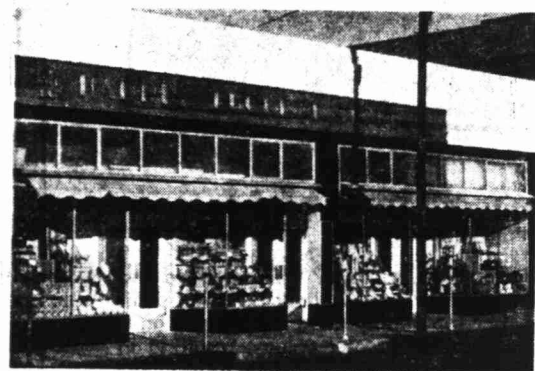
HARRIS-LUCKETT STORE Air Conditioning by Neill's Sheet Metal Co.
