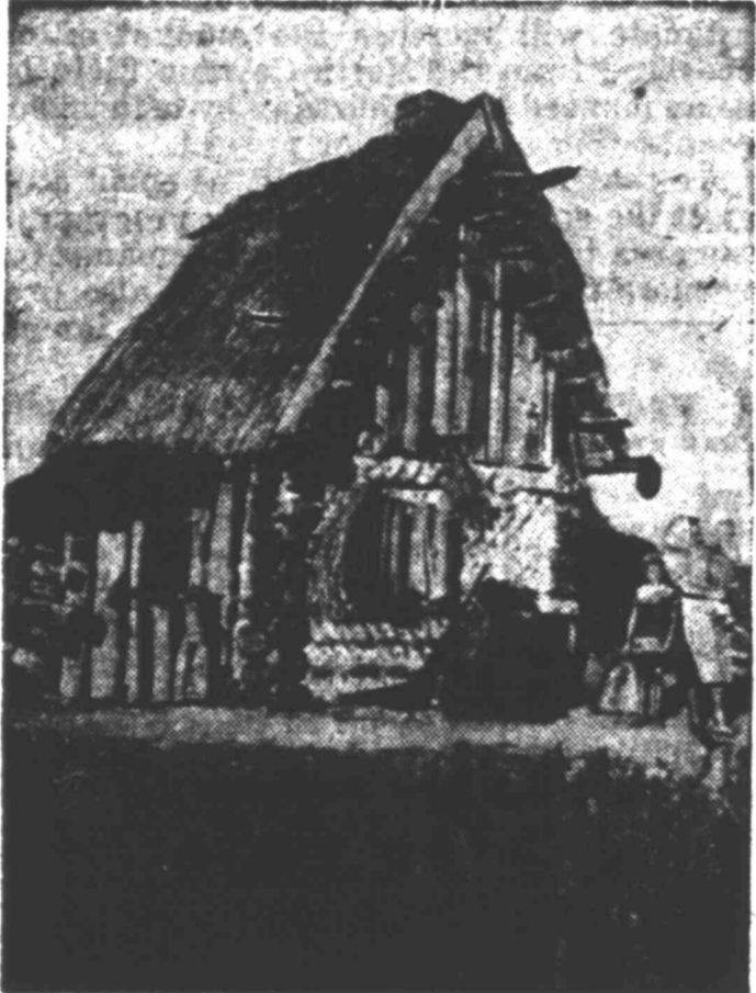
Farm family's home in a devastated region, built of salvaged wood and grass thatch.
