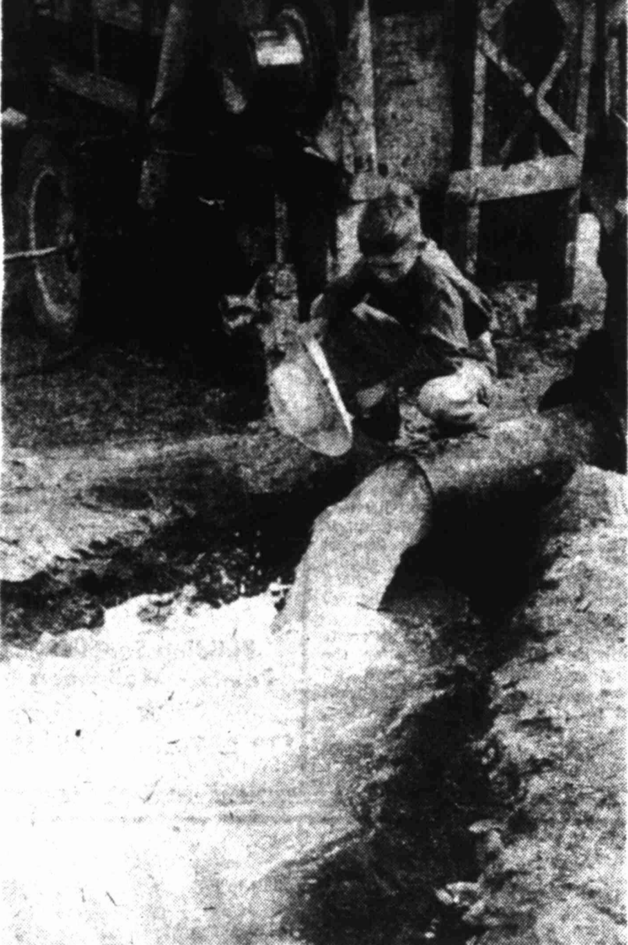
James Barron, son of Mr. and Mrs. Elliott Barron, watches water gushing at the rate of 900 gallons per minute from a well recently completed on the M. F. King ranch about eight miles northwest of Midland. The well made this amount of water on a 24-hour test. Charles Barron, son of Mr. and Mrs. T. Paul Barron, took the picture.
