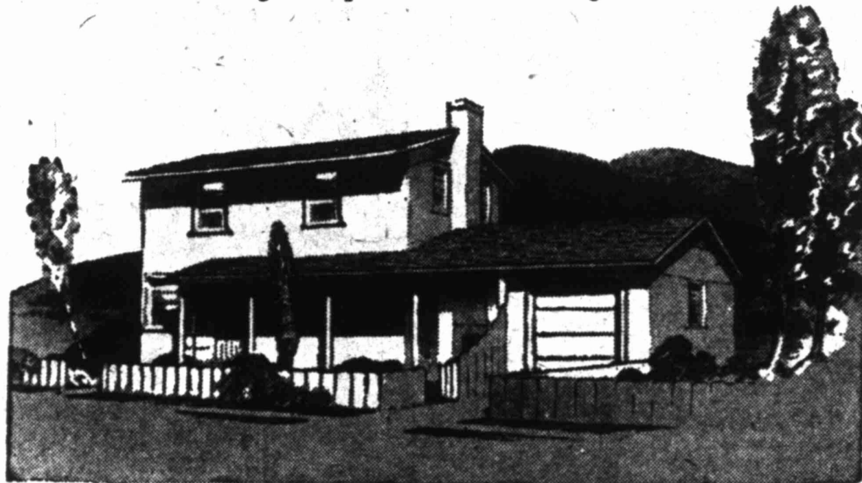
This attractive and delightfully livable dwelling is an Industry Engineered home which saves cost of material and labor by utilizing standard measurements. Such homes allow individuality and beauty of design while aiming at economy in construction costs. The measurements are in multiples of four inches. The attractive exterior of this modern dwelling is exceeded only by the beauty and comfortable living qualities of the complete and well arranged interior.
