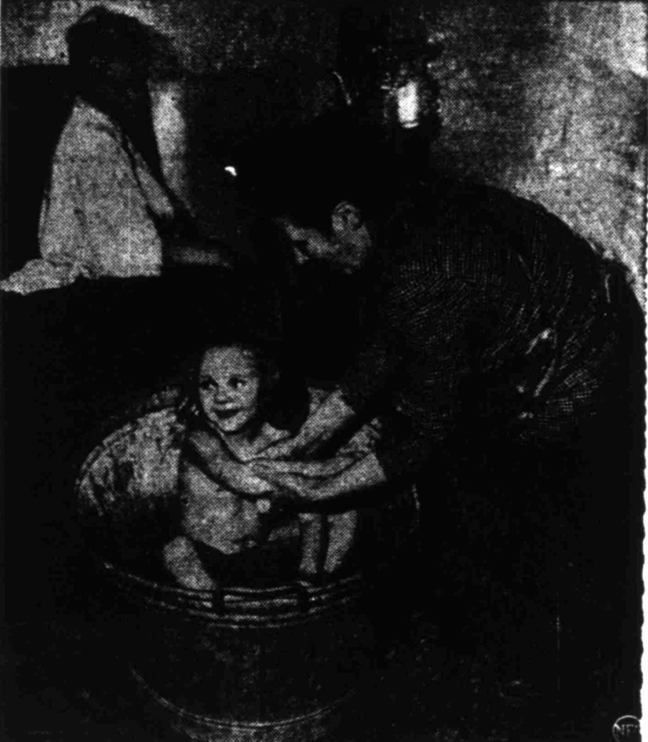
Hot water is precious—so the children receive a hot bath only once a week in this tub in the von Schmudes living room.
