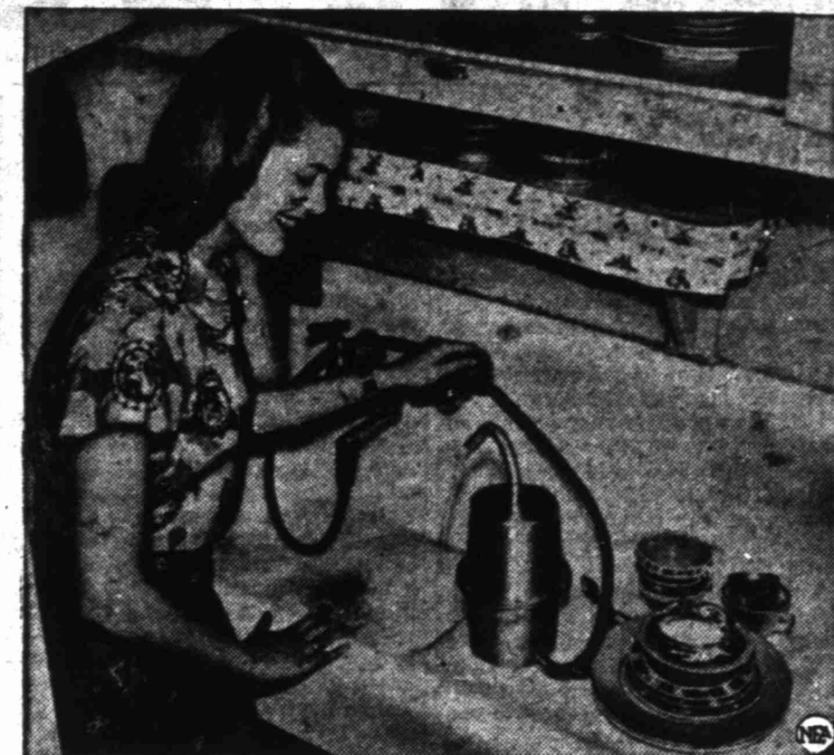
Free flow of water through this small-scaled aluminum water softener is made possible by non-clogging glass fiber screens in the container. Hose which hooks softener to faucet is detachable.
