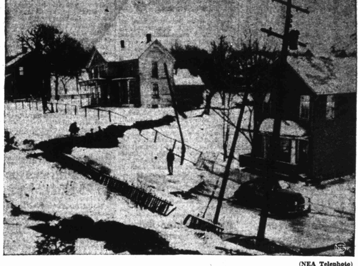
Kane Street in Carbondale, Pa., sags more than 20 feet after the collapse of an underground anthracite mine shaft. Four persons were injured and 14 homes were damaged by the collapse. A warning rumble preceded the cave-in, waking residents and enabling them to escape.
