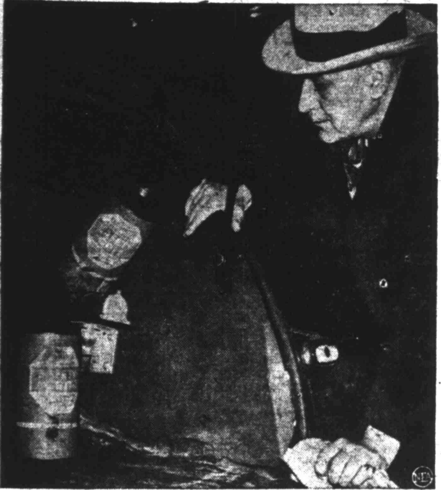
Chairman of the Chicago Traffic Commission, inspects a new traffic safety device to prevent skidding on slippery pavements. The operation is similar to the sanding of slick rails by a locomotive engineer. Abrasive traction material is carried in two
