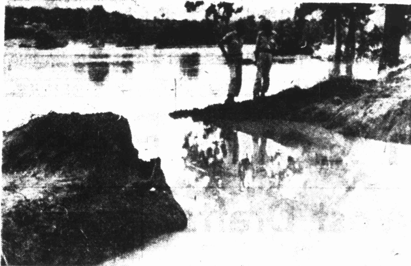
(NEA Telephoto) Before construction crews could repair damaged levees on the Trinity River at Fort Worth, fresh rains put the river up to the 13-foot stage and water started filling the lowlands along the river where the levees still were broken. The flood passed without any major damage.
