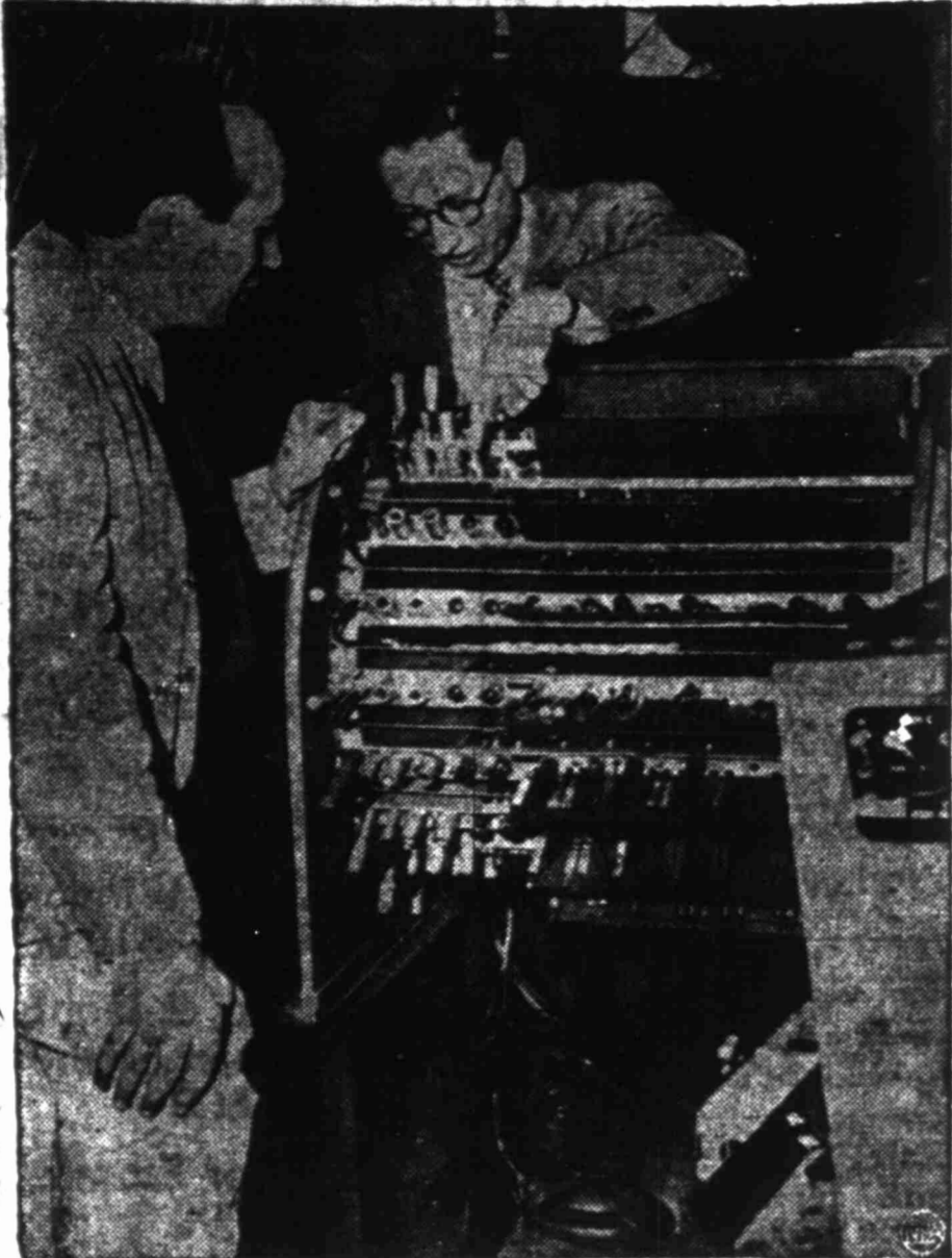
The portable "electronic brain" above, called Binac, can solve mathematical problems 12,000 times faster than a human brain. Its co-designer, J. Presper Eckert, Jr., left, and James R. Weiner, right, chief engineer, look over their brainchild in Philadelphia. Besides solving complicated engineering problems, Binac can work out military strategy, compose music and play chess. For something like $250,000, you can buy one to do Junior's homework.
