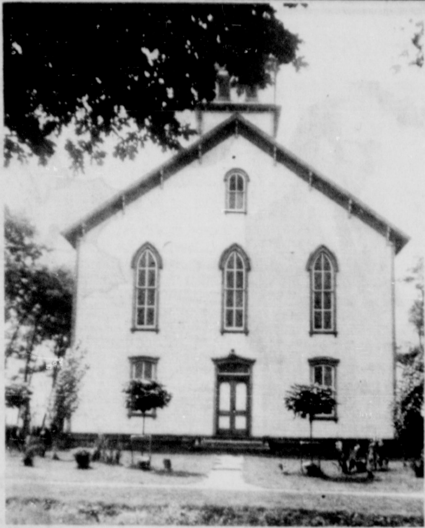
BUILDING STILL STANDS.... This rural Presbyterian Church building still stands near West Lebanon, Pennsylvania, where Mabel Cunningham DeLong grew up. Activities here played a very important part in her life during her growing-up years. She says, "The lower floor was occupied by Sunday School rooms and worship services were conducted in the upper story."
