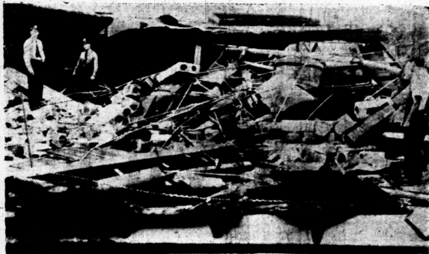
(NEA Telephoto) Cars are pinned under the wreckage of a plastic mould factory in South Easton, Mass. The town was hit by a strong wind of tornado intensity which blew down the factory killing one and injuring many.
