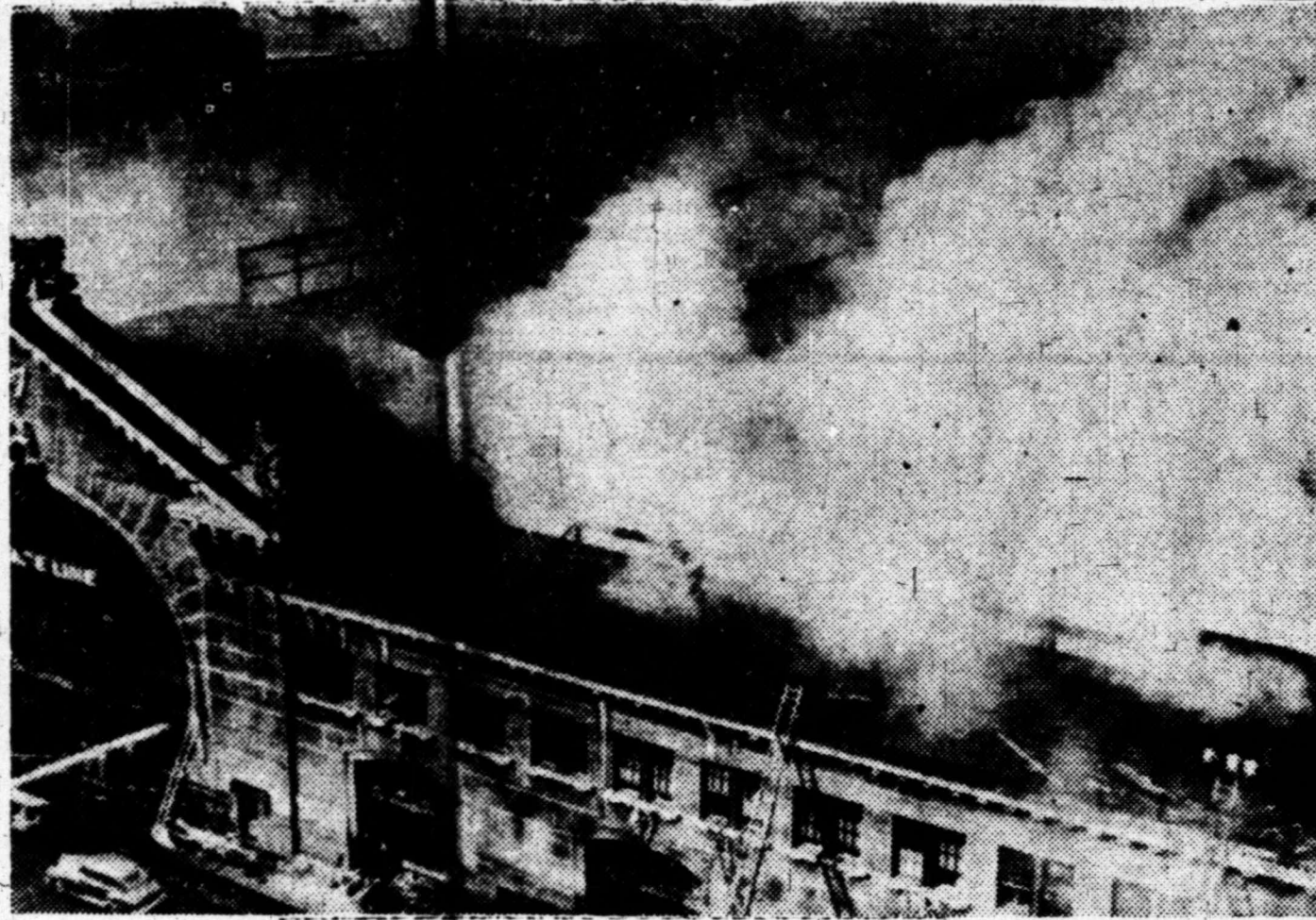
Early Monday morning fire broke out on Gotham Pier, on the Hudson River. Five alarms were sounded in Manhattan and three in Brooklyn. Thick, black, oily smoke poured hundreds of feet in the air. The pier was destroyed. (NEA Telephoto)
