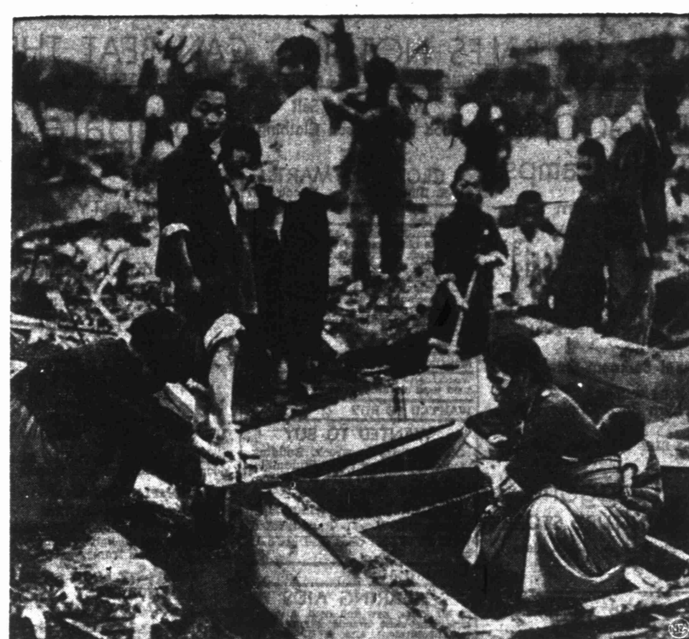
SO YOU THINK YOU HAVE A HOUSING PROBLEM? — There's no day nursery in war-blasted Wonsan, Korea, to park baby while mama gets on with her task of rebuilding their wrecked home. So this Korean lady, strapped to its mother's back, gets a rough ride as she helps her companion saw up part of the house frame for rebuilding.
