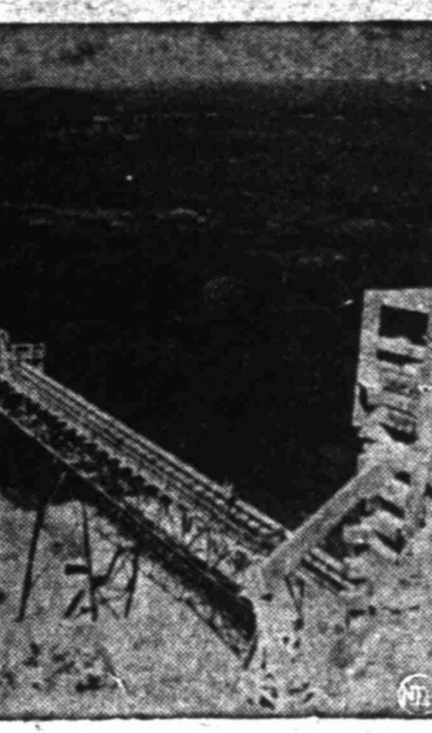
Mountain on the move—Seven-mile belt conveyor winds through the Ozarks to carry four million tons of Lee Mountain across two valleys to the site of the Bull Shoals Dam.
