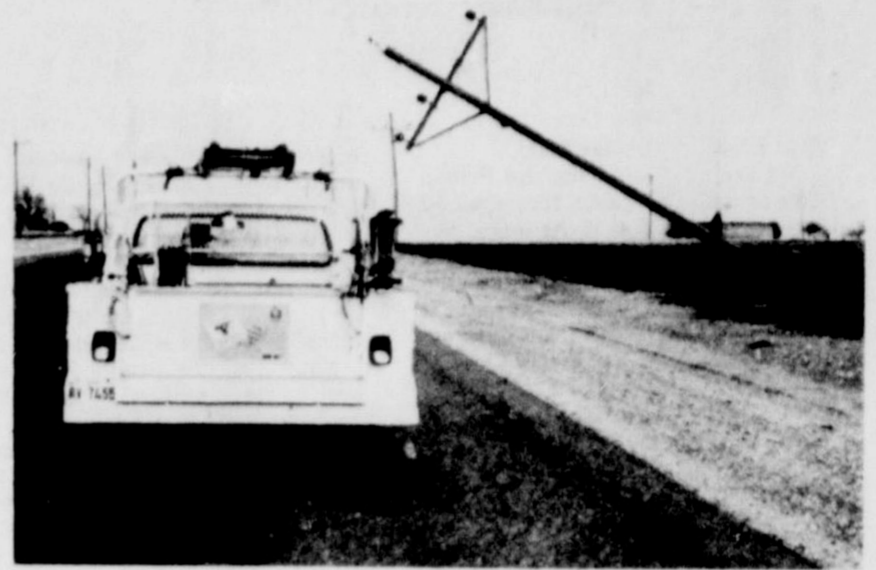
POLE BROKEN.... So strong was the high wind of Tuesday, that a utility pole was snapped just off Highway 214 south of Friona. An
