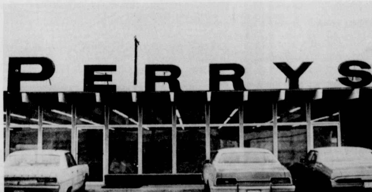
NEW STORE....The exterior of the new Perry's store, which opened on Friona's North Main Street Friday morning, is shown above. Perry's has completely re-modeled the building, which formerly housed Piggly Wiggly super market, and installed carpet. The store kicked off a grand opening sale, advertised on Pages 8-9.
