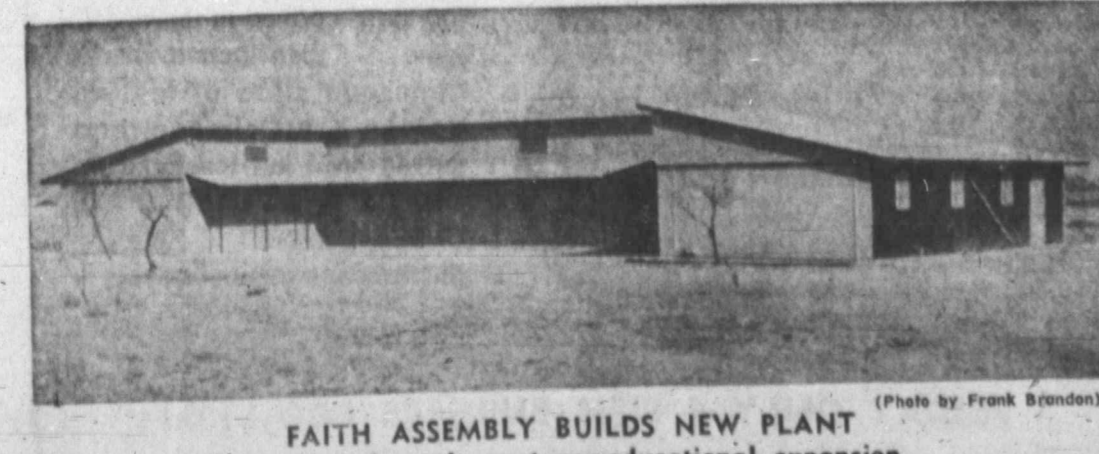
FAITH ASSEMBLY BUILDS NEW PLANT Part of a planned sanctuary-educational expansion
