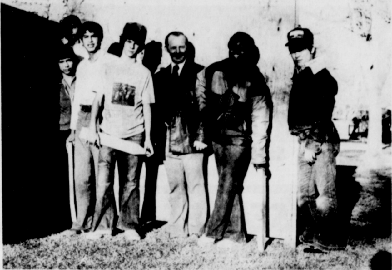
SANTA'S HELPERS.... Members of Friona Junior High School's CVAE building trades class have been working to build a "Santa's Workshop" in the City Park this
