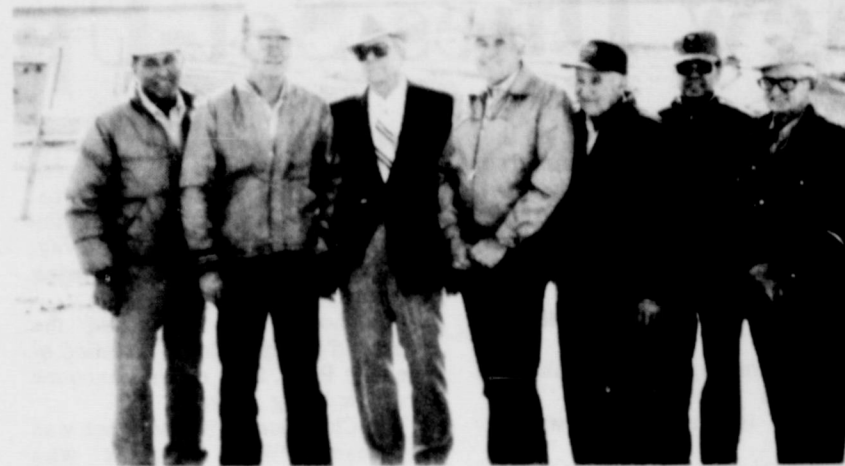
TAKE TOUR....Touring the Lazbuddie Flood Prevention Dam during a final completion check were, left to right, Don Ramsey, SCS construction engineer; Raymond McGehee, County Commissioner; Paul Fortenberry, County Judge; Jack Patterson, County Commis-
