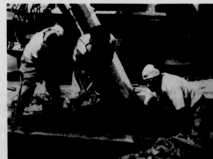
HIGHWAY WORK... Workmen are shown putting in a new drive entrance at the Tasty Cream location on Highway 60. Work continues on removal of the medians and replacement of curbs and gutters through the city.
