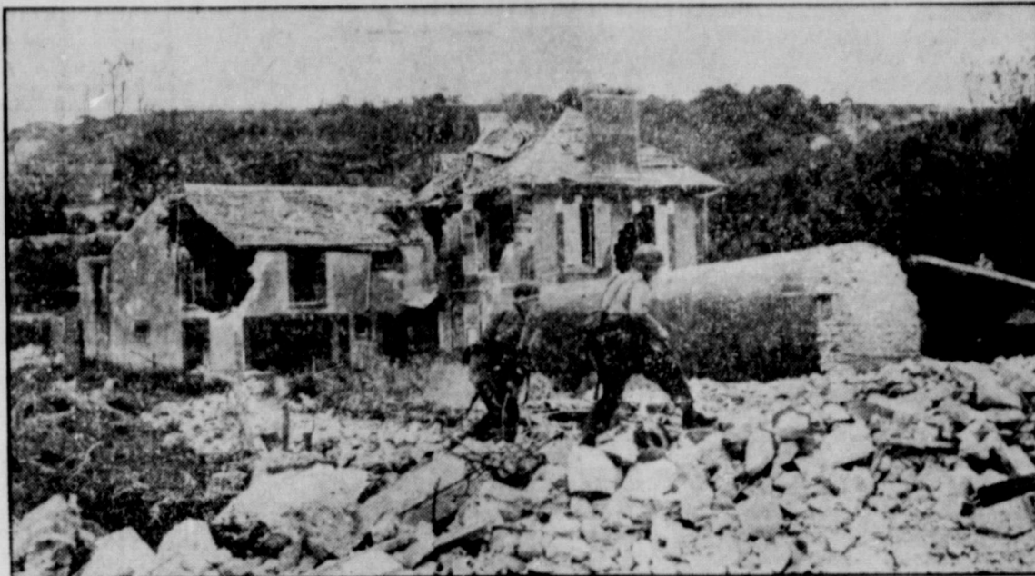
This house in a small village in Normandy was used as a fortress by the Nazis, who added refinement of a concrete road block. Allied guns blasted their work to rubble.
