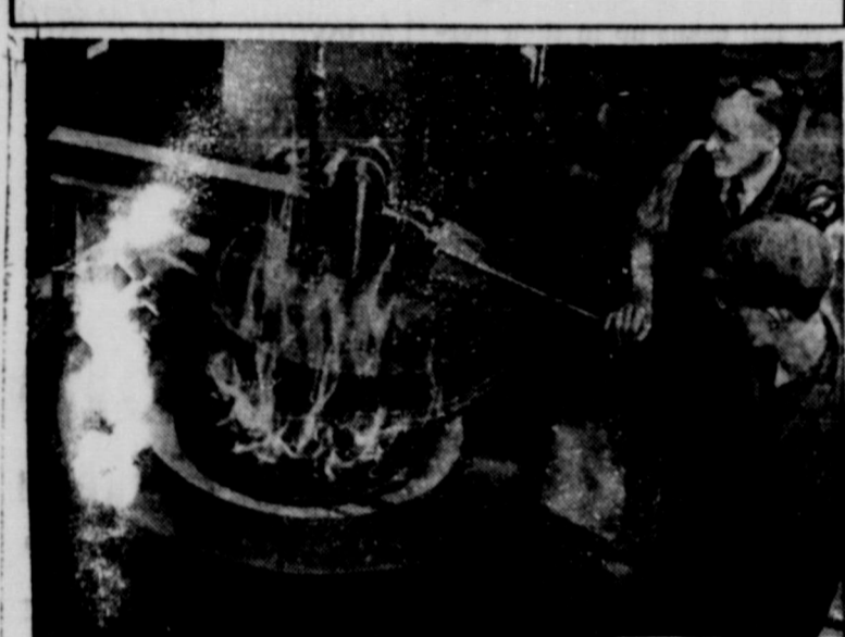
Metal aircraft fittings are removed from heating furnace and dipped in oil bath. Treatment increases life-span of metal, is vital wartime contribution.
