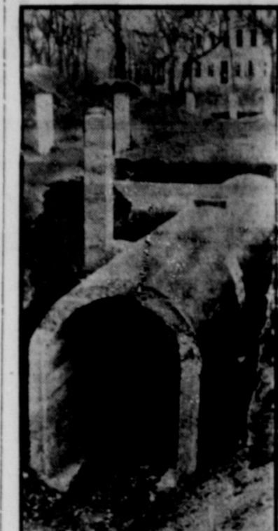
This is one of the air attack shelters in Coblenz, where civilians lived for days at a stretch. It winds on back toward the building in the background, with ventilation shafts showing at intervals.
