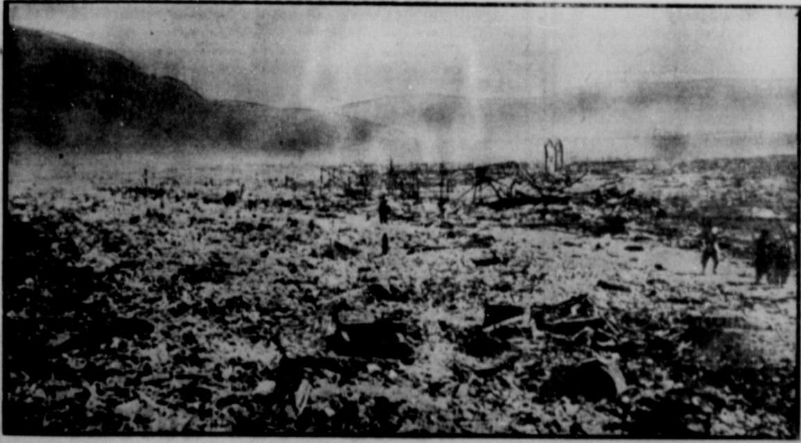
Just a few steel girders remain upright where the atom bomb landed and flattened Nagasaki, second Jap city to feel its awesome scourge. This was a factory district in the city of 210,000.
