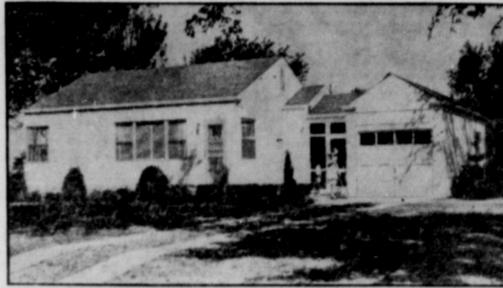
Aluminum houses like this Butler Boulevard Aluminum Home shown at Kansas City, Mo., are one of the newer creations designed to relieve the housing shortage. The house, 24 feet by 33 feet in overall dimensions, can be put up in two and a half weeks. Home contains 2300 pounds of steel, mostly in roof and rafters.
