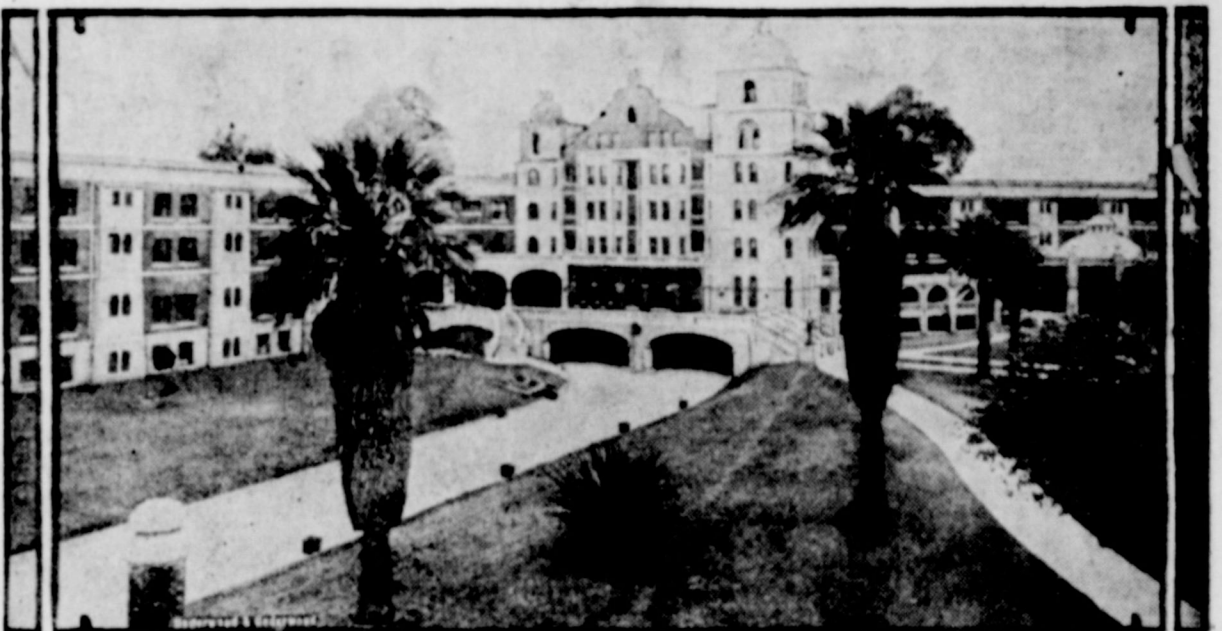
The famous Arlington hotel at Santa Barbara, Cal., that was wrecked by the earthquake shocks which destroyed much of that city. Photograph by courtesy of the Rock Island railroad.
