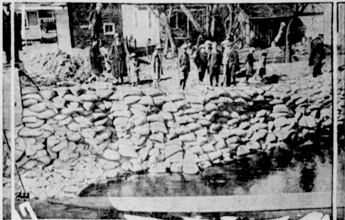
After an all-night fight, residents of Portage, Wis., succeeded in blocking a break in the wall of a canal between the Fox and Wisconsin rivers, and saved the town from an imminent flood. The high waters forced down seventy-five feet of the wall, and weakened the gates at the Wisconsin river end of the canal. Citizens filled the gap with granite and sandbags.
