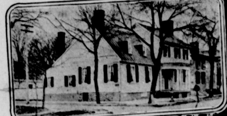
MARY WASHINGTON HOUSE, FREDERICKSBURG, VA.
