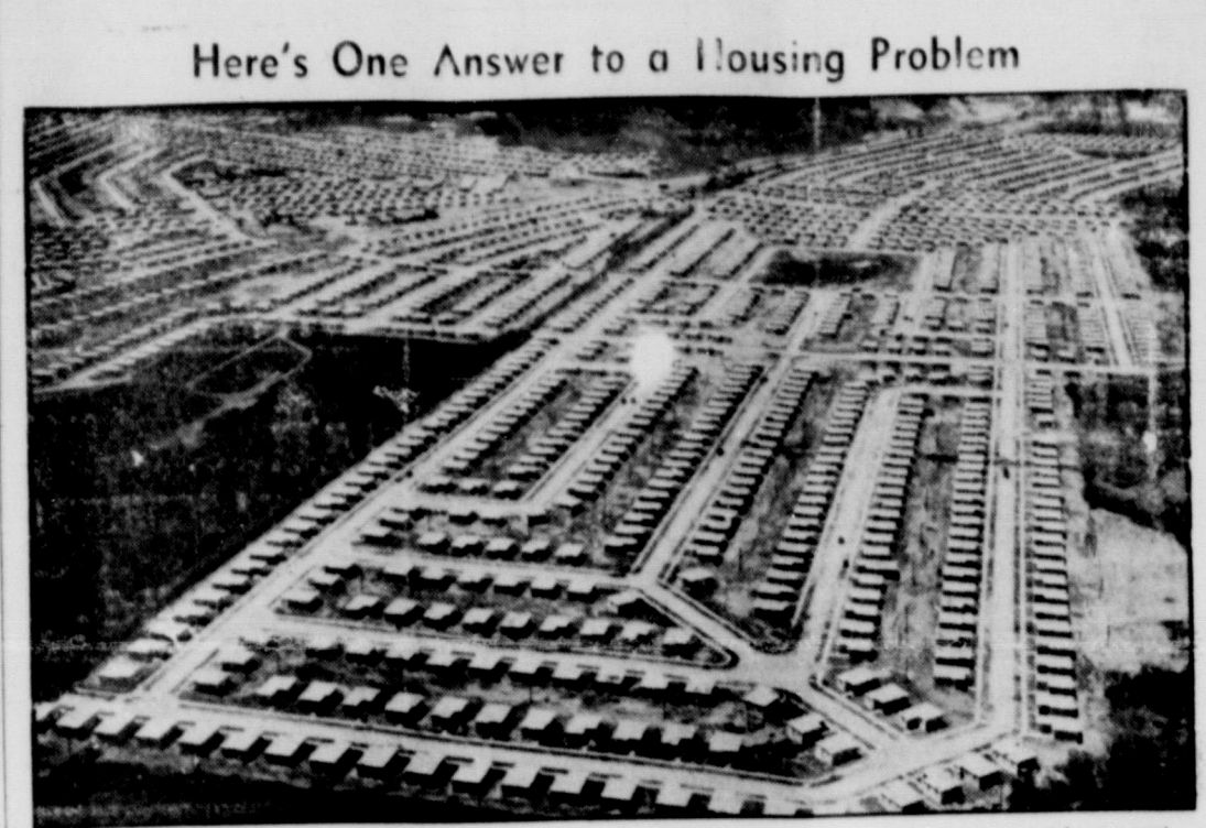
Here's One Answer to a Housing Problem Nearing completion five miles from San Juan, capital of Puerto Rico, is one of the world's largest private housing developments, Puerto Nuevo. Above are some of 3500 concrete, five-room dwellings built in slightly more than a year's time, with 1500 others soon to be completed. They sell for an average of $4000 and were constructed by a South Carolina builder in co-operation with the FHA and Puerto Rico government to alleviate the island's acute housing shortage.
