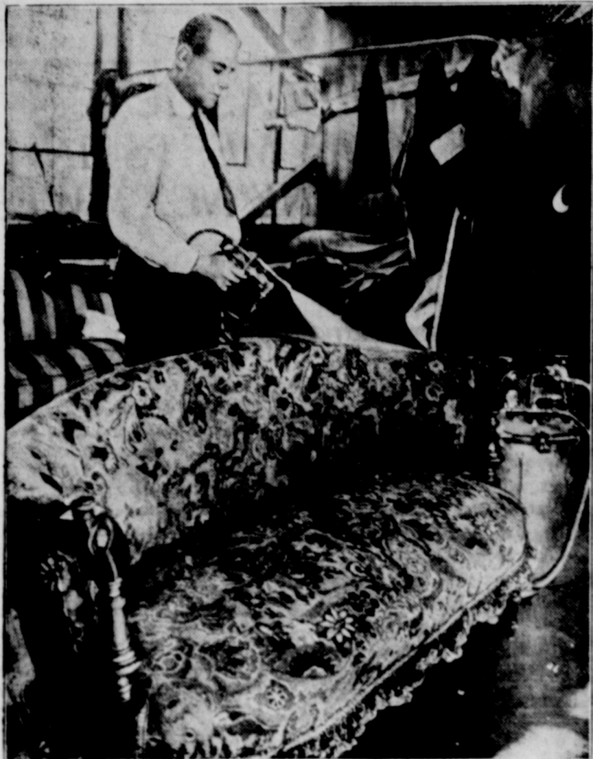
Using Air Pressure to Apply an Aqueous Fluoride Solution to Moth-Proof Wool Tapestry.
