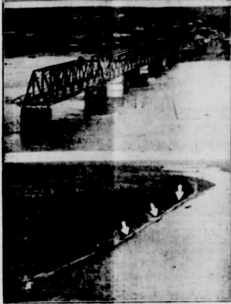
The top photo is a closeup aerial photo of the bridge over the Rio Grande River showing how the middle spans were washed away by debris piling up against them as the muddy waters swept towards the sea. Below is a section of the Southern Pacific tracks near Del Rio, inundated by the Rio Grande.
