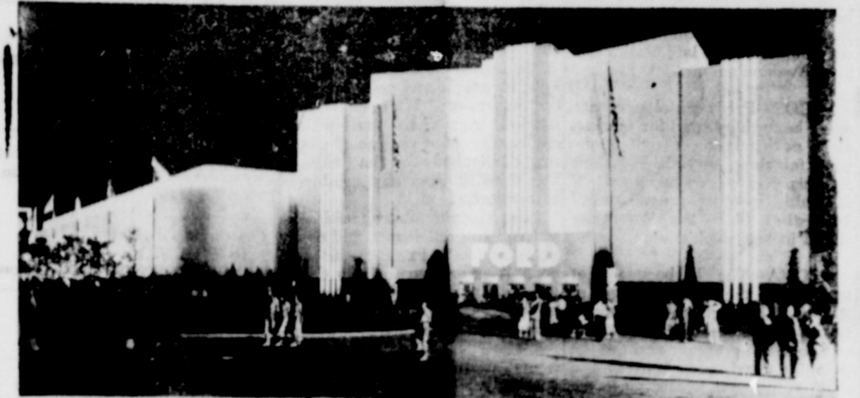
Its solid white walls flooded with many lights, the huge Ford Exposition building at the Texas Centennial in Dallas makes an attractive and imposing structure at night. Parapet lighting adds beauty to design. The front of the building, which faces Federal Concourse, has rows of Neon tubing which contribute much to the general lighting arrangements.
