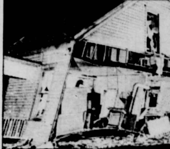
GONE WITH THE WIND . . . Most of Belleville, Ill. was just that after tornado killed eight, injured scores and cost $1,000,000; this demolished home is typical of damage.
