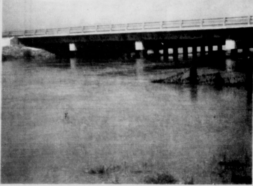
LOTS OF WATER was running under this bridge on Running Water Draw between Bovina and Farwell. This is the fastest the water has been sweeping down the draw in many years.
