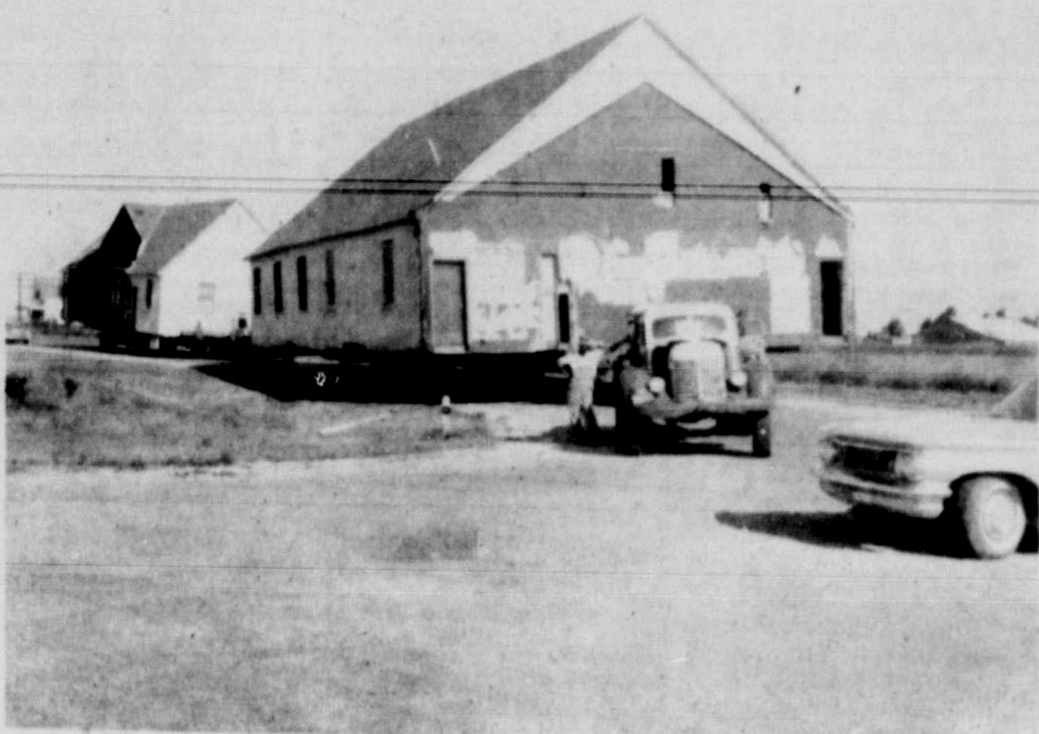
A PRETTY GOOD LOAD---One of the largest house moving projects around Friona lately took place Saturday when movers picked up what is to be the new home of the Calvary Baptist Church over in Bovina and began their way to Friona. The two-piece church building is shown above at the intersection of Highway 60 and the Rhea road awaiting REA personnel to drop power lines so they can move to their destination north of town.
