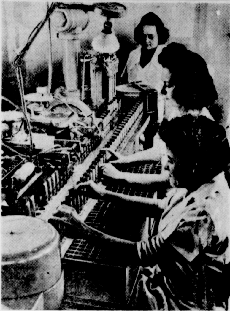
At the Whitehall Pharamcal Company in New Haven, Conn., empty toothpaste tubes are inserted into the automatic machine which fills, closes, crimps and seals them. In this industrial process, as in thousands of others, used cooking fat substitutes for industrial fats and oils that can not yet be imported from the islands of the South Pacific.
