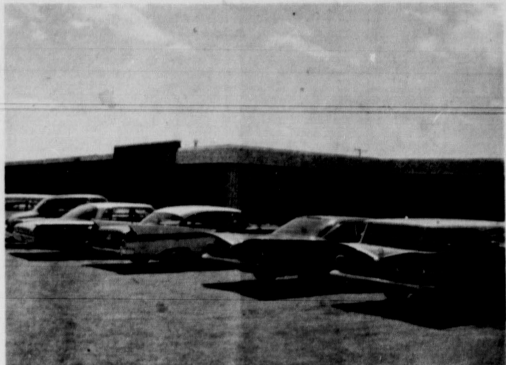
HOSPITAL ADDITION--A view from the northeast corner of Parmer County Community Hospital shows the new addition to the building. Open house is planned April 9.
