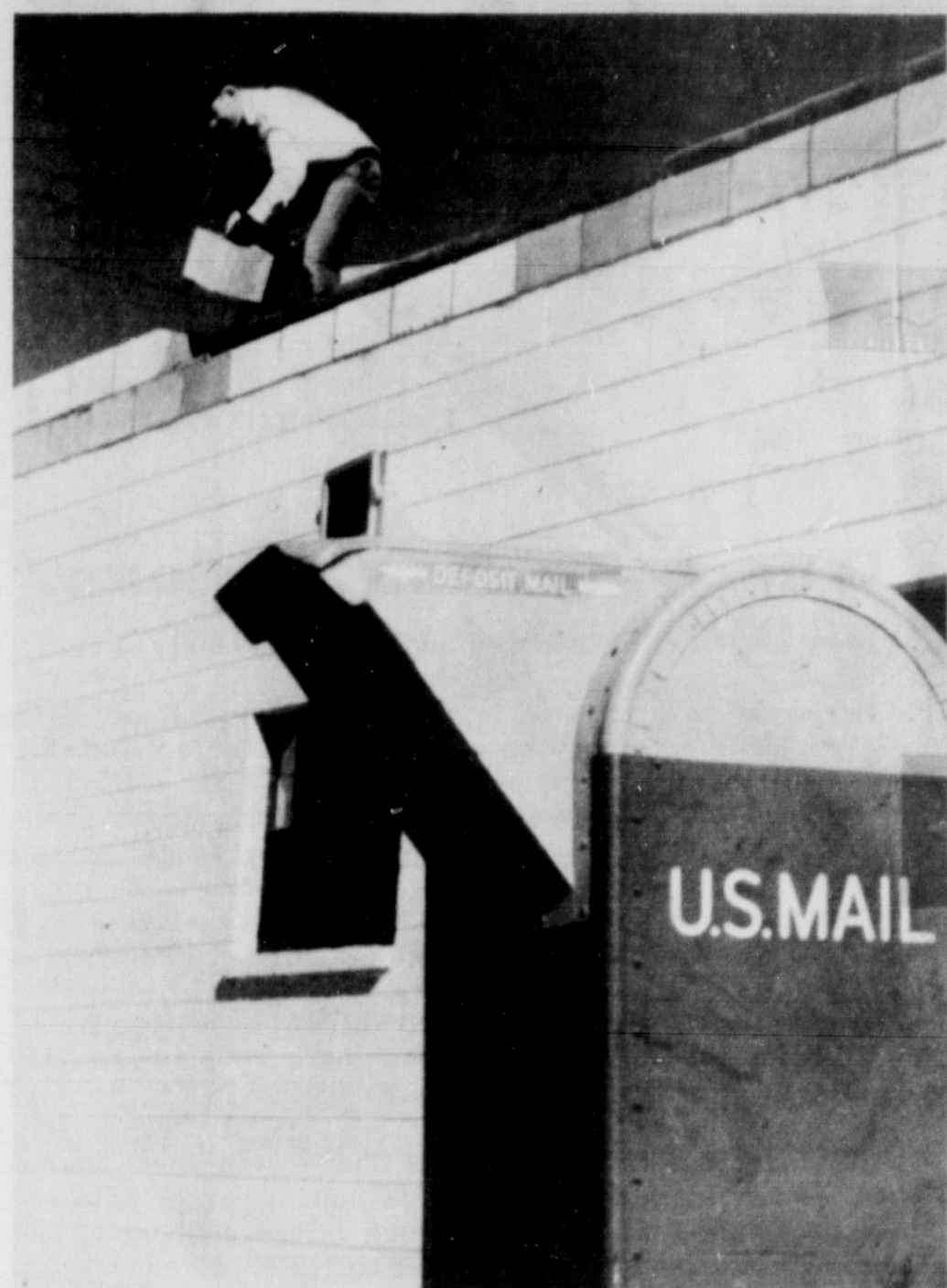
A NEW CROWN... A workman places new tile around the top of the post office building after a transport truck caught the low-hanging telephone wire and pulled out part of the east wall. The top layers of tile were replaced around the building last week.
