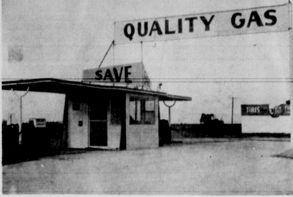
THIS PORTABLE SERVICE STATION is Friona's newest business and it is scheduled to open this week end. The new station, located in the east part of Friona on Highway 60, was built and installed by the Portable Service Station Corporation of Hereford. The station was built of steel and it is the fourth one to be completed and installed by the corporation. Other stations built by the firm have been located in Utah and Colorado. Carl Moseley of Hereford says that the station will be leased, but that he will probably run it himself at the present time. A grand opening is planned later.
