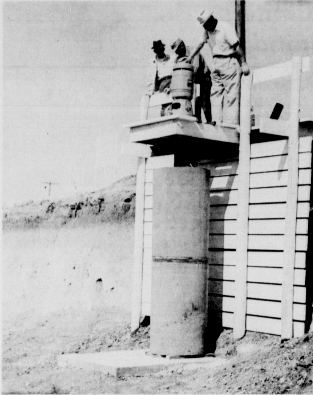
HELPING INSTALL a tailwater pump system on the James Mabry farm at Hub are these representatives of the High Plains Water district. This pump is to be a special test case in that it is designed to filter out weed seeds and other material which sometimes causes problems in tailwater pump operations.
