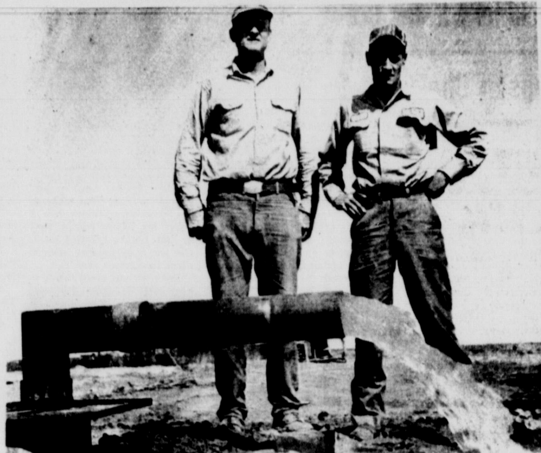
Left to right are Eulis Waggoner of Dimmitt and O. D. Scheller, owner and operator of O. D.'s Pump and Machine Shop of Earth. The water is 350 feet down and being pumped up by this 40 horse power motor.
