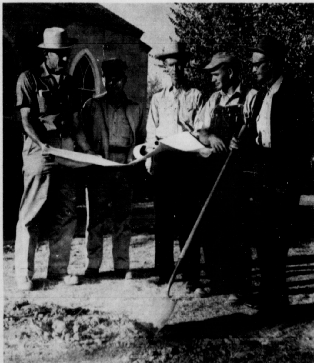
BREAKING GROUND . . . Members of the Tenth Street Church of Christ are shown with George Taylor (left) as preliminary dirt work was begun for the church's new building this week. From the left are Taylor, Edgar Walters, Calvin Martin, Richard Perkins and A. H. Hadley.
