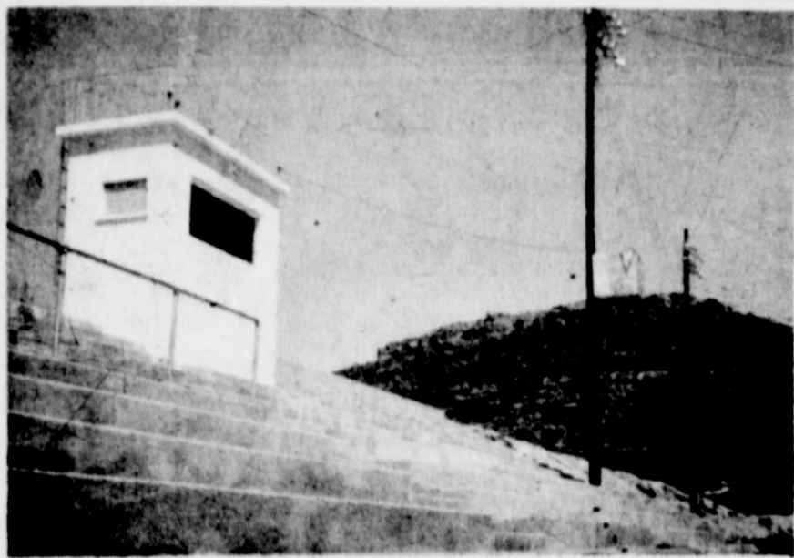
A view of the addition to the seats and the new announcer's booth and photography platform is shown in the picture above. There were five tiers added to the seats on the north side of the football field with the booth on top. The top of the booth has a railing around it and will serve photographers at a vantage point for their work of filming the games.
