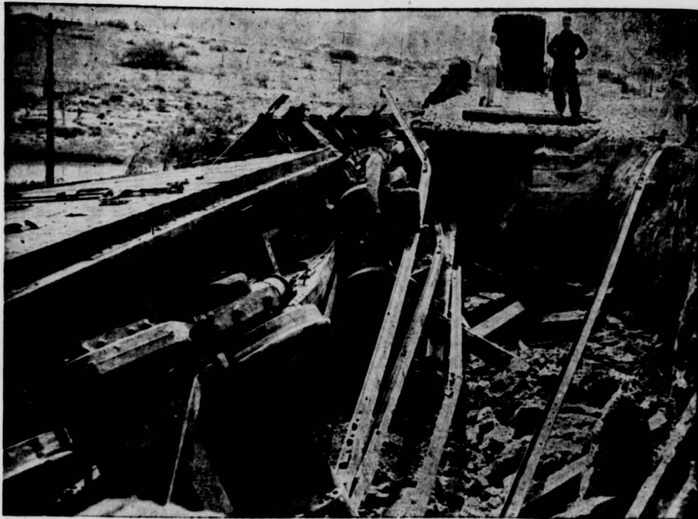
INTO CREEK —Flood waters which swept away the earthen track bed east of Rankin on Monday night plunged three cars of a Santa Fe freight into the waters, derailed seven cars. Standing on top of one of the wheels of an
