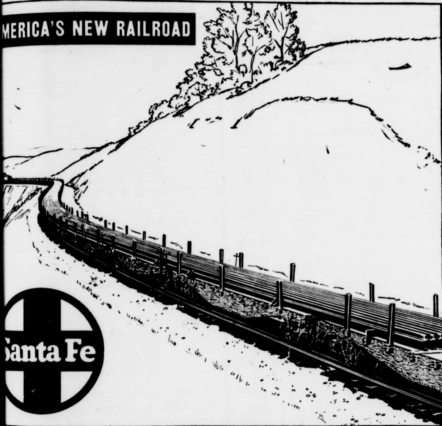
Quarter-mile lengths of welded steel rail curve around a foothill like wire cable.
