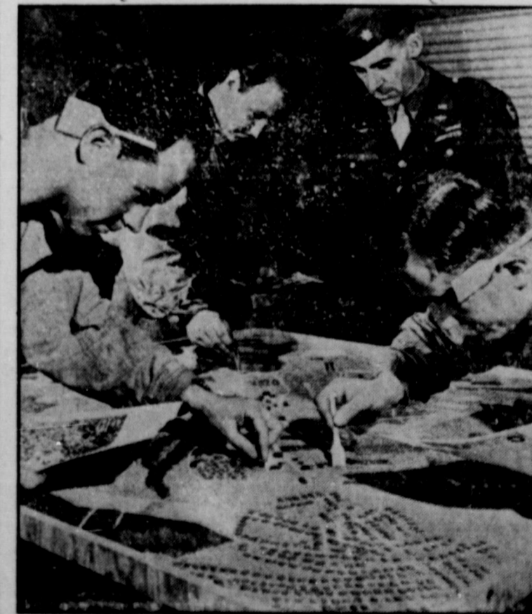
This operation—construction of a scale model of the target, showing each building and the terrain around—precedes Allied bombing operations from England. The models are made from reconnaissance photos, and the flyers study them before embarking to destroy them. Left to right, working on the model, are S/Sgt. Warren G. Gilbert, S/Sgt. Russell Tesmer, and Sgt. Aldo Tonelli, while looking on is Lieut.-Col. Alfred H. von Kolnitz.
