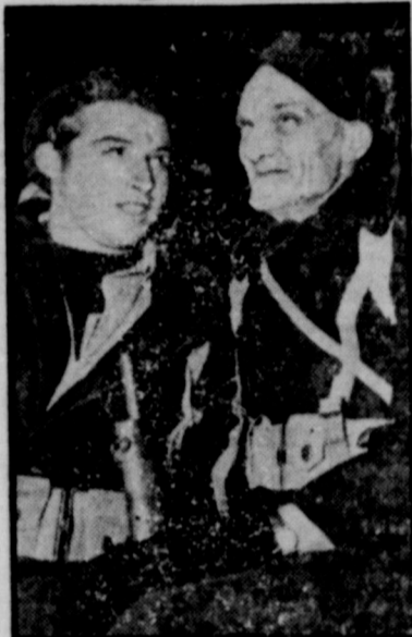
After 10 months "over there," the youngest member of the Navy's 54th Construction Battalion, Carpenter Jim Titherington, 18, left, and Painter Charles L. Bixby, 52, the oldest, are glad to be back. Bixby's got two
