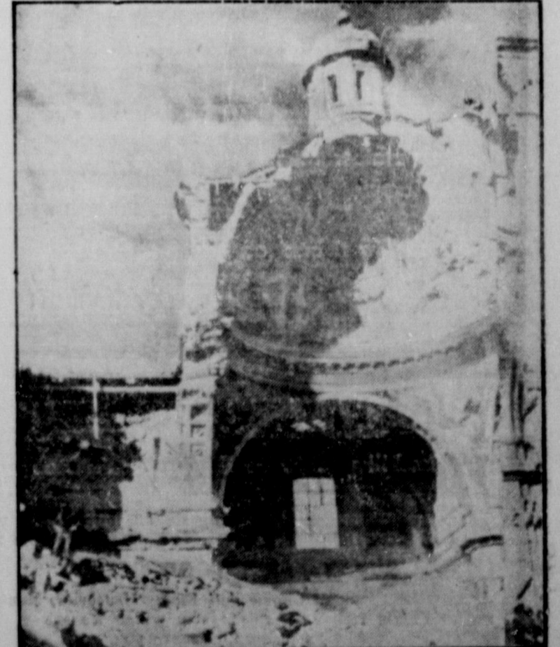
This shows a job done by the fleeing Germans on the 1100-year-old St. Thomas Cathedral in Ortona, Italy, after the Canadians entered the town. Destruction of the church was one of the enemy's last acts, an attempt to impede the advancing Allies. (OWI radiophoto.)
