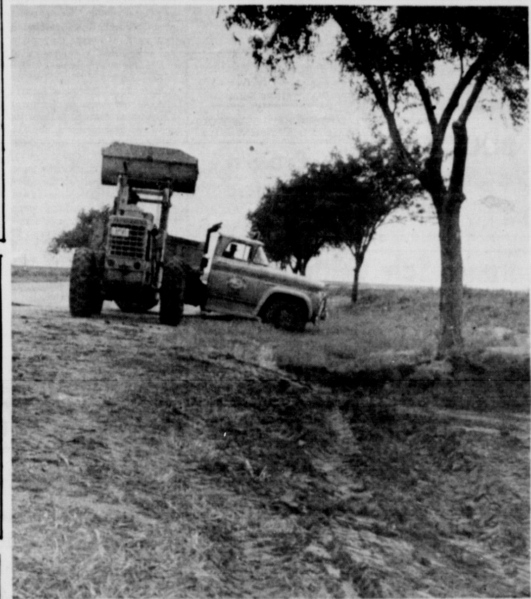
SCOOPING UP loads of what was formerly rich farm land, crews from the Highway Department dug out tons of rich soil from a highway borrow ditch last week. Some farmers were to use the soil for their lawns -- sort of expensive lawn dirt.
