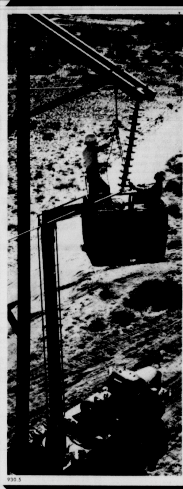
Picture shows an example of modern construction methods. The aerial, truck-mounted bucket lift is being used by two linemen in a safe and efficient manner to construct a new 230,000 volt transmission line.
