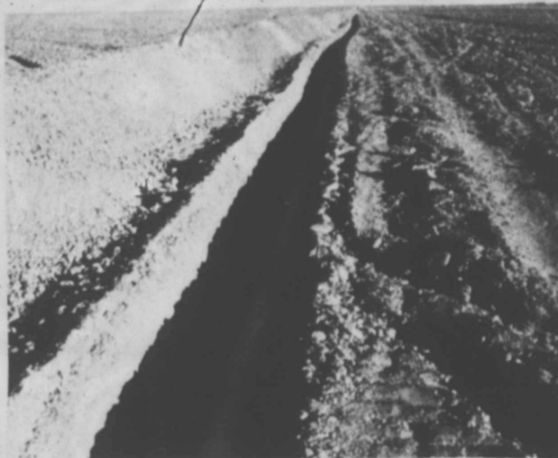
Installation of a high pressure underground irrigation pipeline for sprinkler irrigation system on Coleman Terrell's farm 5 miles east of Sudan.
